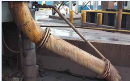
Rotary Vacuum Drum Filter Drain Line
