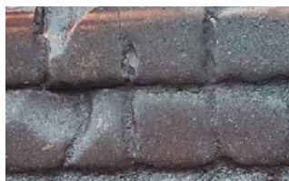
Standard ceramic fracture & joint erosion
