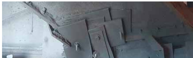
Temporary metal patches
