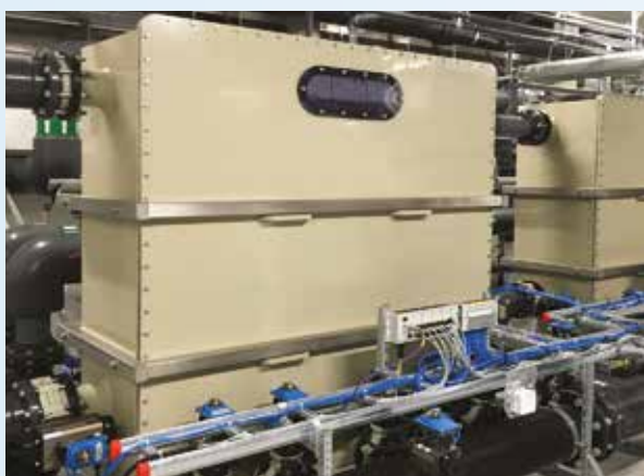
Vacuum mode configuration sports and therapy pools, Norway – 540 m 3 /h
