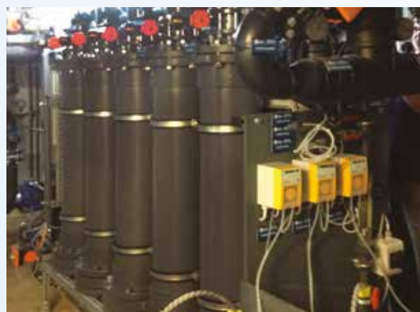
Pressure mode configuration wellness pool, Germany – 80 m 3 /h
