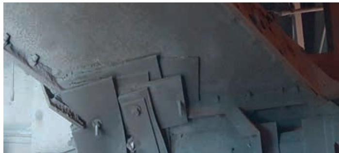
Temporary metal patches
