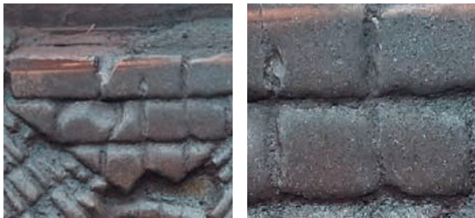
Standard ceramic fracture & joint erosion
