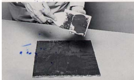
3. Apply adhesive to back and sides of tile
