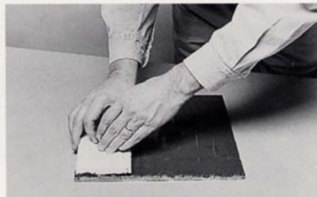
4. Affix tile to surface and press firmly in place
